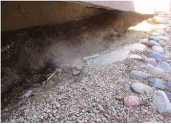
1.3 - Drainage under driveway is blocked on west side with limited flow recommend professional service
