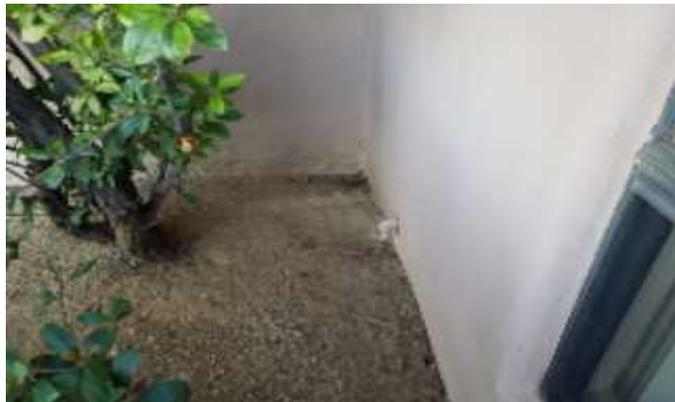
FG water drains and or stands against the structure
