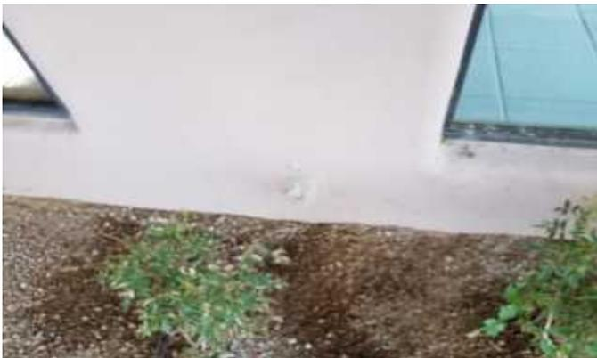
WD water damage to the stucco or sprinkler heads hit it
