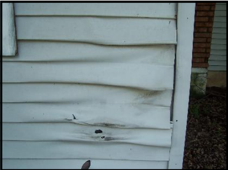
Damaged Siding
