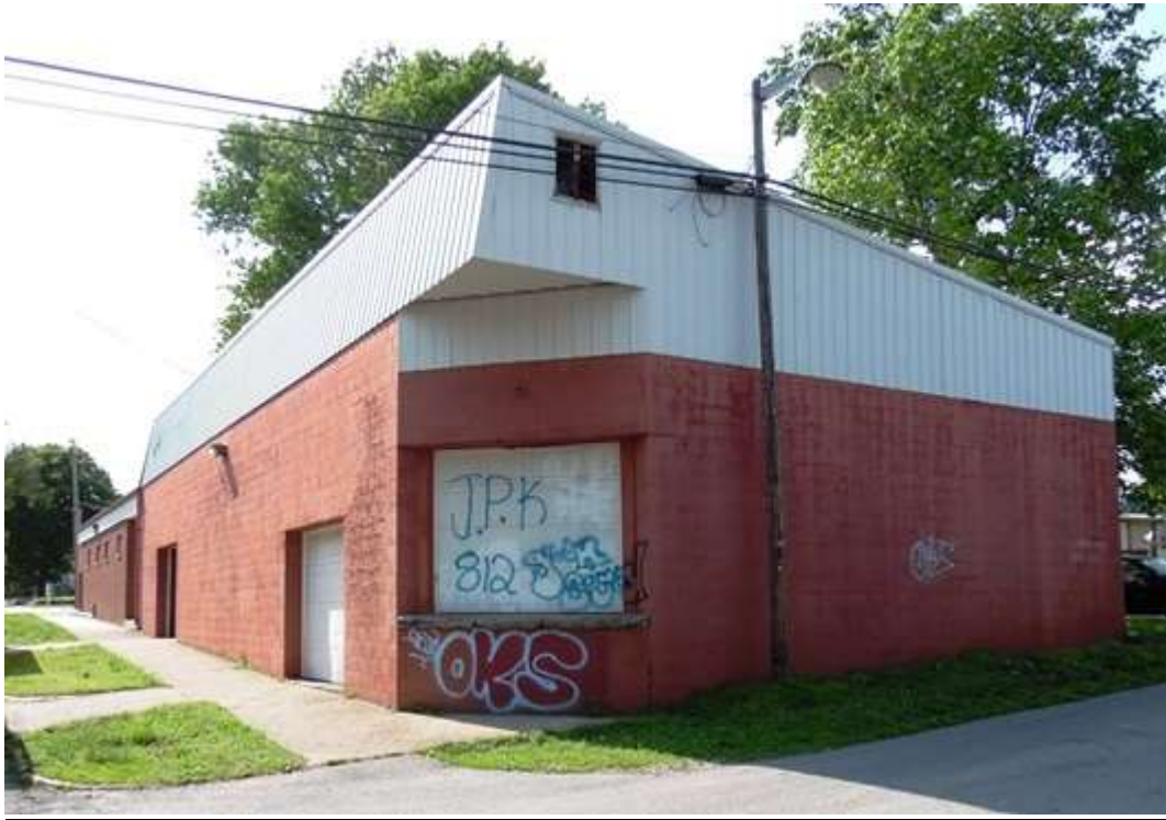
Rear View of 430 & 432 South 7 th Street
