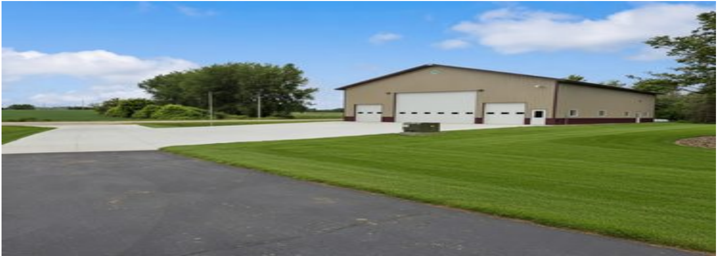
Brand-new 2024 60' × 80' × 18' (4,800 SF) heated post-frame steel shop — high clearance, furnace, multiple overhead doors, bathroom rough-in with shower installed.
