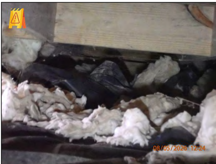
Limited Visual (Entire Front/Right Of Structure)
