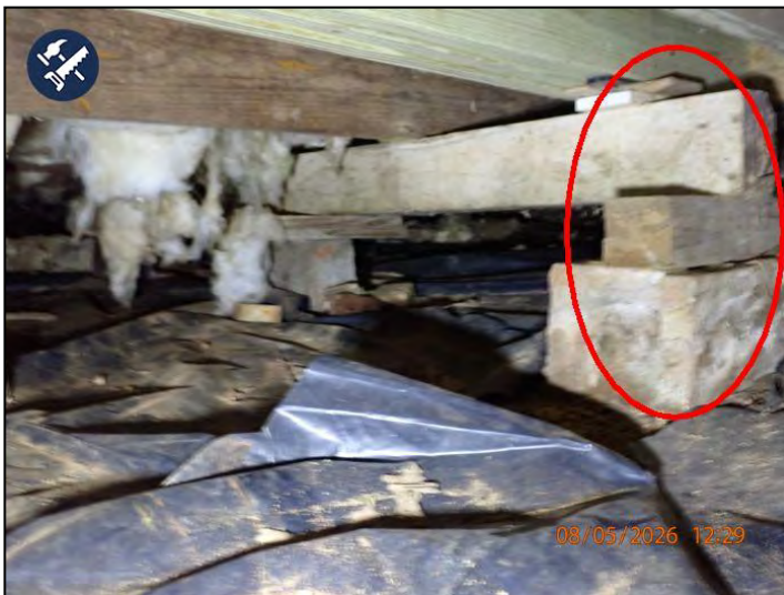
Free Floating Support(s) (Multiple Locations)
