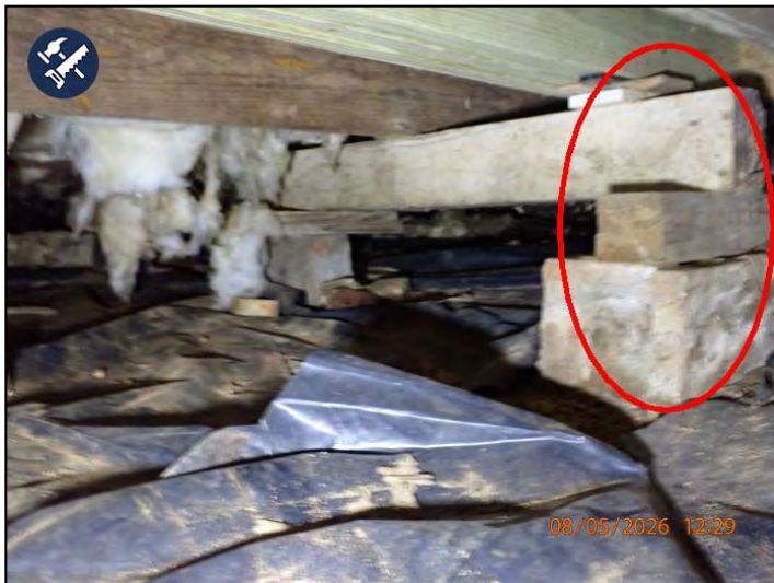
Free Floating Support(s) (Multiple Locations)
