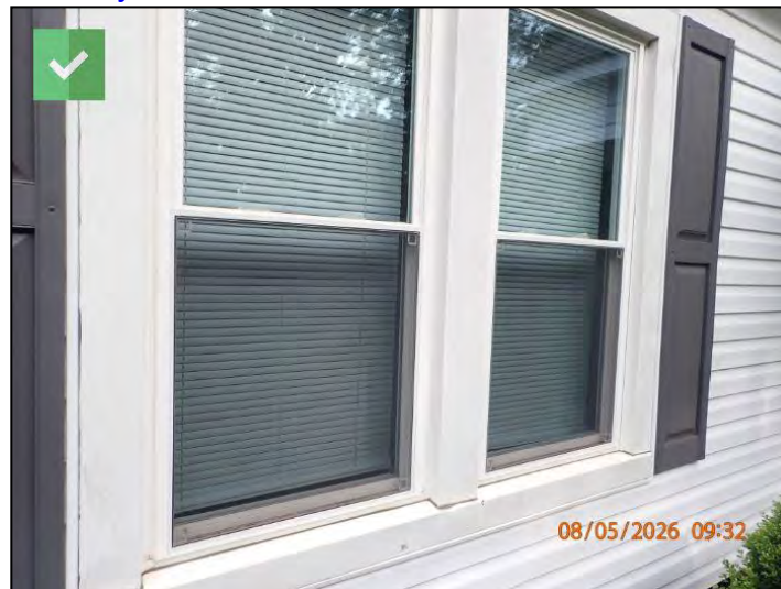
Screens In Place
