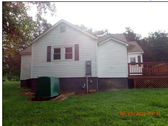
Rear Of Structure
