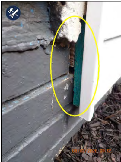
Exposed Wooden Sheathing (Multiple Locations) Exposed Wooden Sheathing (Multiple Locations)
