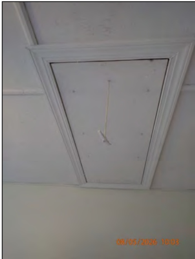
Pull Down Ladder Location: Bedroom #2
