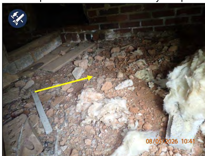
Partially Installed Vapor Barrier
