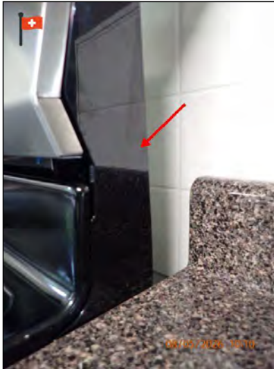
Missing Anti-Tip Bracket
