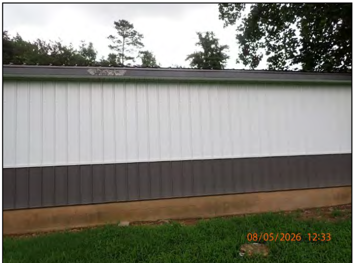
Rear Of Structure
