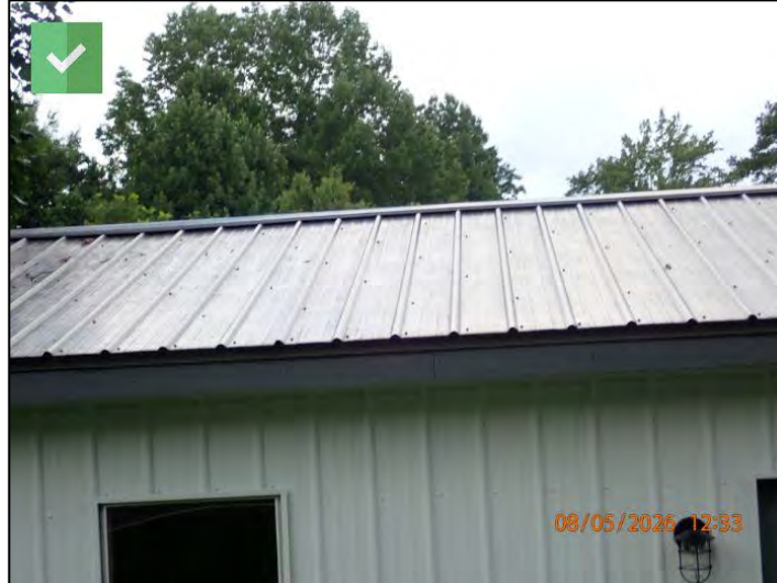
Metal Standing Seamed Roof
