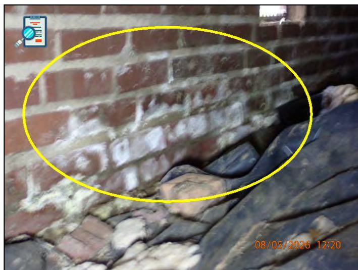
Efflorescence
