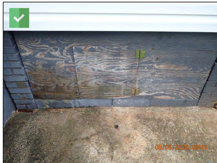
Foundation Access: Rear Of Structure
