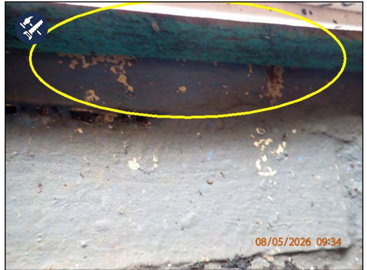
Exposed Wooden Sheathing (Multiple Locations) Exposed Wooden Sheathing (Multiple Locations)
