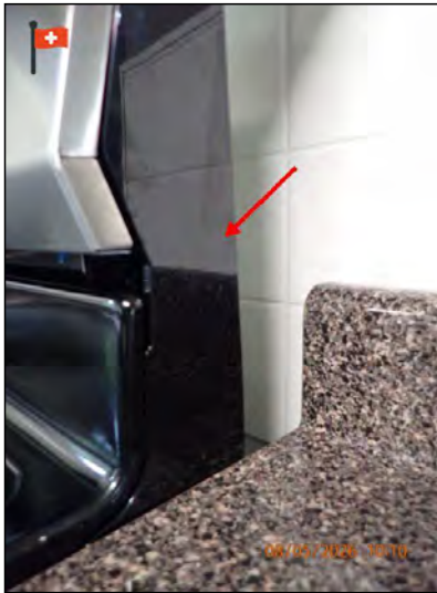
Missing Anti-Tip Bracket
