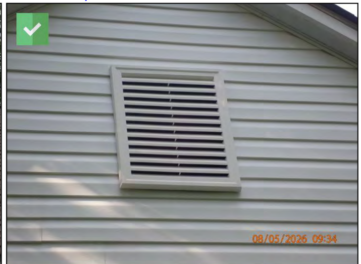
Gable Louver Vents
