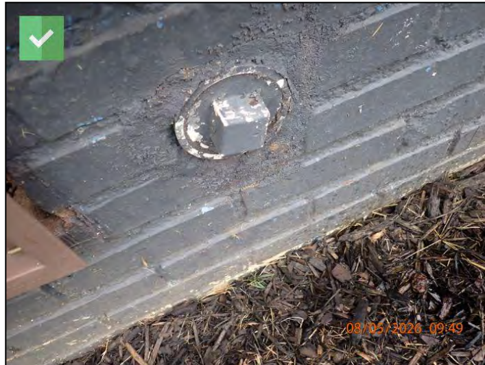
Plumbing Clean Out (Left Of Structure On Foundation Wall)
