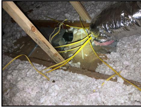
Vents to attic
