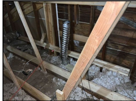
Vents to attic
