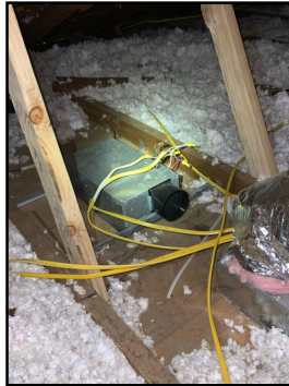
Spliced wires
