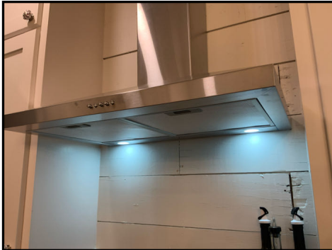
Range hood was functional
