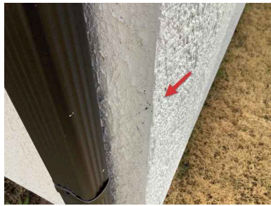
Light coverage at corners around structure
