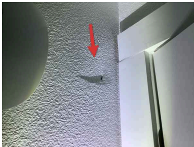
Front storage closet behind door
