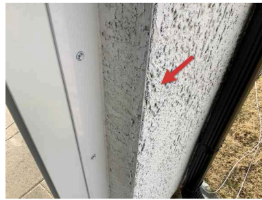
Light coverage at corners around structure
