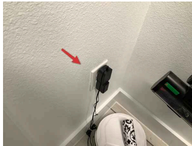
Front storage closet
