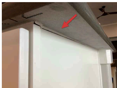
Around Island at countertop to cabinets
