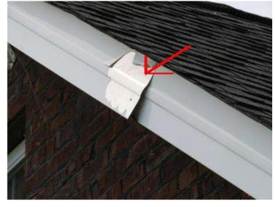
**Maintenance:** Soffit trim noted as loose and hanging in several locations around the structure at time of inspection. Suggest securing.
