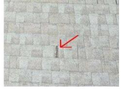
Maintenance: Nails Protruding: This condition can lead to damage to existing shingles and moisture penetration over time. Suggest securing, caulking, sealing nails, nail holes to prevent water entry.
