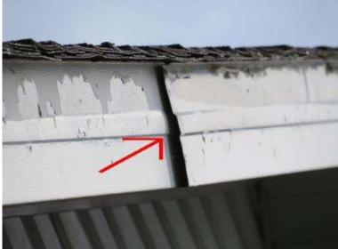
**Maintenance:** The roof ridge boards metal trim at the rear bonus room roof line is damaged / bent and in need of repair or replacement to prevent further damage or loss.
