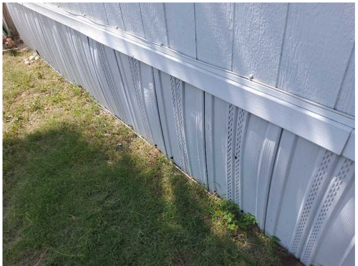
Skirting ( slightly damaged small holes weed eater damage)
