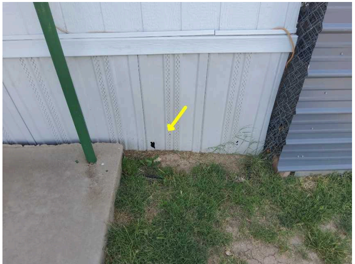
Skirting ( slightly damaged small holes weed eater damage)
