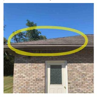
4.4.3 Insufficient number of downspouts for size of roof. Install additional downspouts to encourage proper drainage off roof and away from house. **(Various)**
