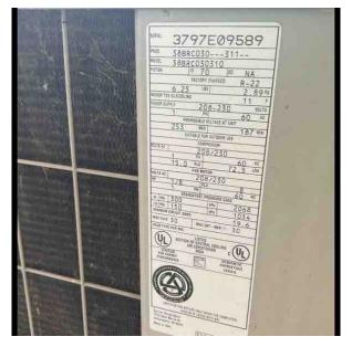
10.5.3 The air conditioning system is past its typical life expectancy. Replace the system when it fails, when repairs are no longer cost effective, or pro-actively to prevent loss of functionality. (Exterior Back)
