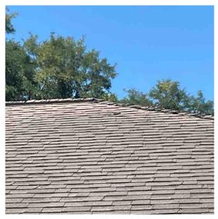
4.2.2 The main house roof covering condition is consistent with what is expected at the first 1/3 of its life. Ask seller to provide warranty paperwork and installer contact information.
