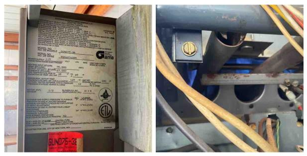
10.6.4 Both the forced air furnace are past the typical life expectancy. Replace the system when it fails, when repairs are no longer cost effective, or pro-actively to prevent loss of functionality.
