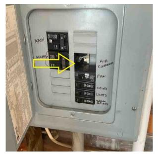
9.7.2 The sub-panel has double-tapped breaker(s). Recommend an electrician further assess and correct as required for electrical safety. (Detached garage)
