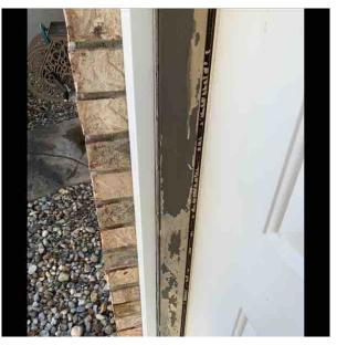
3.4.2 Door flashing is loose. Seal to protect from water related damage. (Detached garage exterior front )
