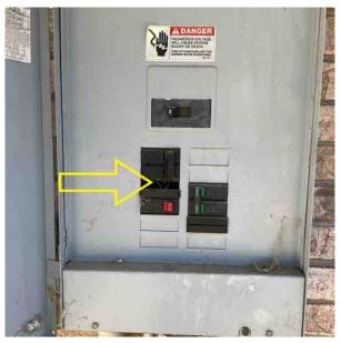
9.5.2 Main disconnect not labeled. Label disconnects for ease of identification and safety. **(Exterior Back)**
