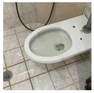
11.9.3 The toilet is loose. Repair as required to prevent water damage. (Bathroom)
