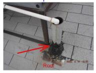
9. Patio Roof Roof Surface Penetrations: Metal Pipes with Tar Flashing - (a) No jack on penetration. (b) Gaps and loose flashing at the HVAC ducts. A qualified licensed contractor is recommended to inspect this system, evaluate all findings, make recommendations and estimate repairs.
