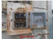
18. \*Sub Panel #1 Location: Patio Area - The neutrals and the ground wires are required to be connected to separate busses in a sub panel. A qualified licensed contractor is recommended to inspect this system, evaluate all findings and estimate repairs.
