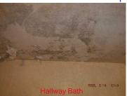
27. All living areas and garage Living Space Interior Floors: Carpet, Tile Floors - Heavy wear throughout the home. Common grout line damage. Missing or deteriorating grout. Recommend re-grouting and sealing the lines. Broken tiles found. A qualified licensed contractor is recommended to inspect this system, evaluate all findings and make any necessary repairs.
