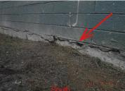
2. Wall Structure: Block, Wood Frame - (a) South: Heavy cracking with displacement noted. Cracking extends into the stem wall. (b) Other Areas: Common cracking and mortar decay noted. A qualified licensed contractor is recommended to inspect this system, evaluate all findings, make recommendations and estimate repairs.
