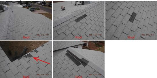
8. Main Roof Roof Surface Penetrations: With Metal Roof Jacks and Caps - Sealant cracking and decayed. Gaps are present at the penetration, this can allow for moisture to enter the home. A qualified licensed contractor is recommended to inspect this system, evaluate all findings, make recommendations and estimate repairs.
