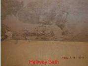
Other, Defective Interior Floors: Carpet, Tile Floors - Heavy wear throughout the home. Common grout line damage. Missing or deteriorating grout. Recommend re-grouting and sealing the lines. Broken tiles found. A qualified licensed contractor is recommended to inspect this system, evaluate all findings and make any necessary repairs.
