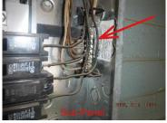
19. Branch Circuit Conductors: Copper Wire 110 VAC circuits - Non-metallic sheathed cable - (a), Exposed wiring present. All wiring needs to be covered, in the wall, or inside proper conduit. (b), Cloth coated wiring is still present in the home. This is aged and should be tested for proper viability and latent damage. A qualified licensed contractor is recommended to inspect this system, evaluate all findings, make recommendations and estimate repairs.
