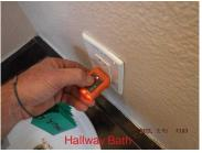
16. Polarity & Ground of all: Exterior & Interior - #1 Bathroom: Open grounds found at the outlet. This location should also be GFCI protected once wiring is corrected. A qualified licensed contractor is recommended to inspect this system, evaluate all findings, make recommendations and estimate repairs. Noted: Single center light on tester indicates open ground.
