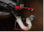
25. All Bathrooms Bathroom Tub/Surround: Porcelain tubs with tile surrounds - Hallway Bath: Heavy rust damage. A qualified licensed contractor is recommended to inspect this system, evaluate all findings, make recommendations and estimate repairs.
