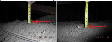
30. Master Bedroom Closet Attic Estimated "R" value. R10 or less - (a) The insulation appears to have 'settled' and would not meet typical standards of the time of construction(8 inches/R-30). (b) IECC standards adopted in 2015 recommend 10 inches(R-38) depth of insulation for Climate Zone 2 areas such as Maricopa and Pima counties in Arizona. Adding insulation to the attic areas if one of the most effective
