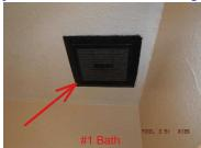
27. Interior Service Area Laundry Room/Area Ventilation: Electric ventilation fan - Fan inoperative. A qualified licensed contractor is recommended to inspect this system, evaluate all findings, make recommendations and estimate repairs.
