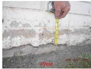
2. Water Penetration or Condensation: Evidence of moisture penetration was found - A qualified licensed contractor is recommended to inspect this system, evaluate all findings, make recommendations and estimate repairs.
