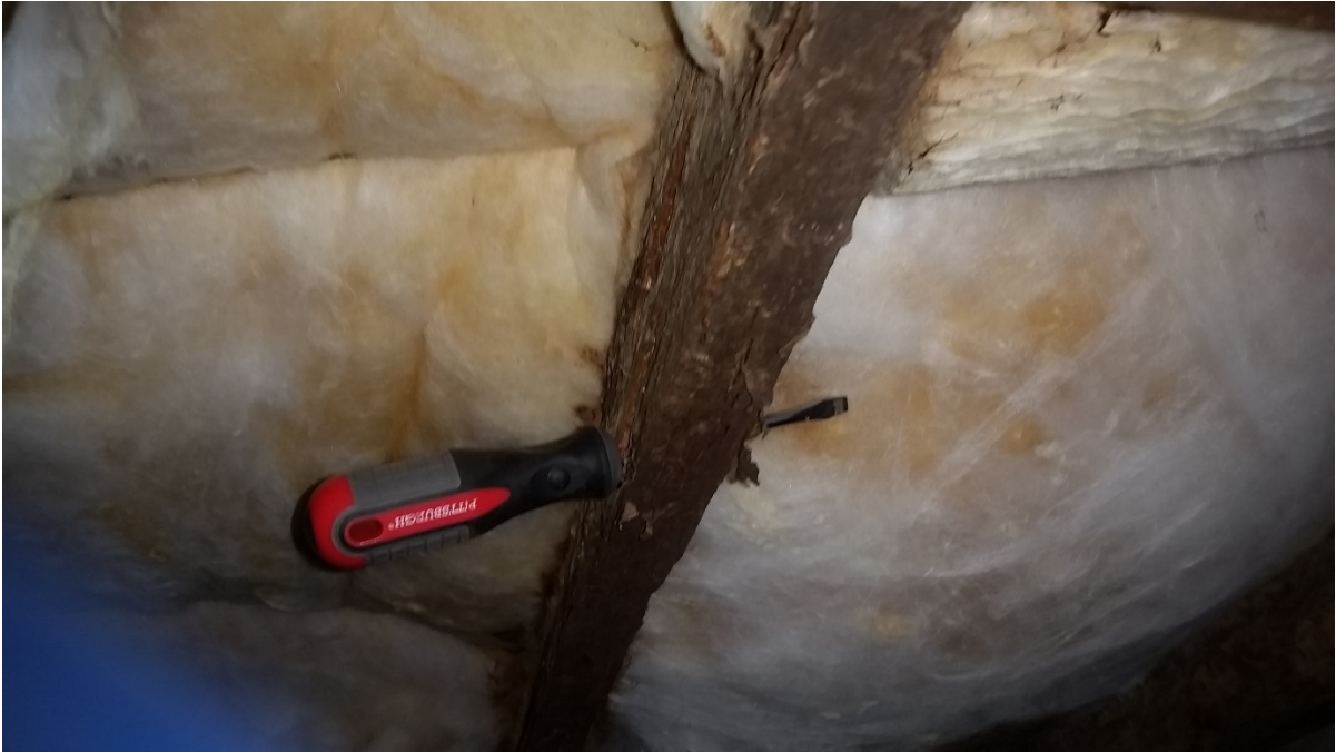
Deteriorated Floor Joist
