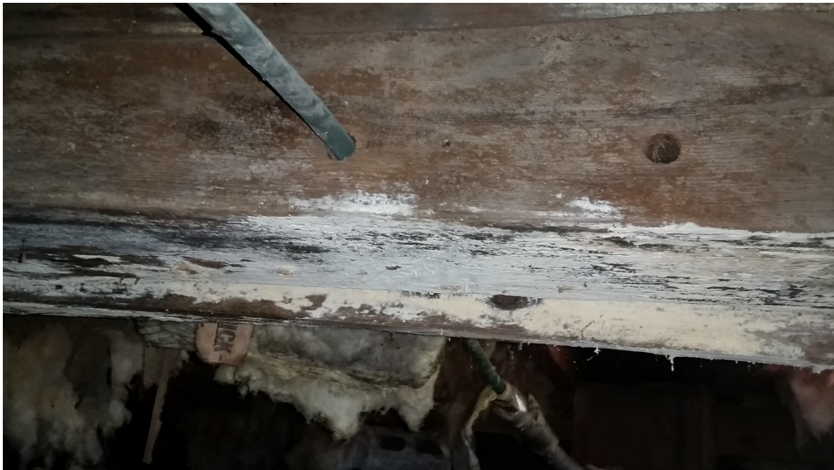
Dark Stains and Mildew on Floor Framing
