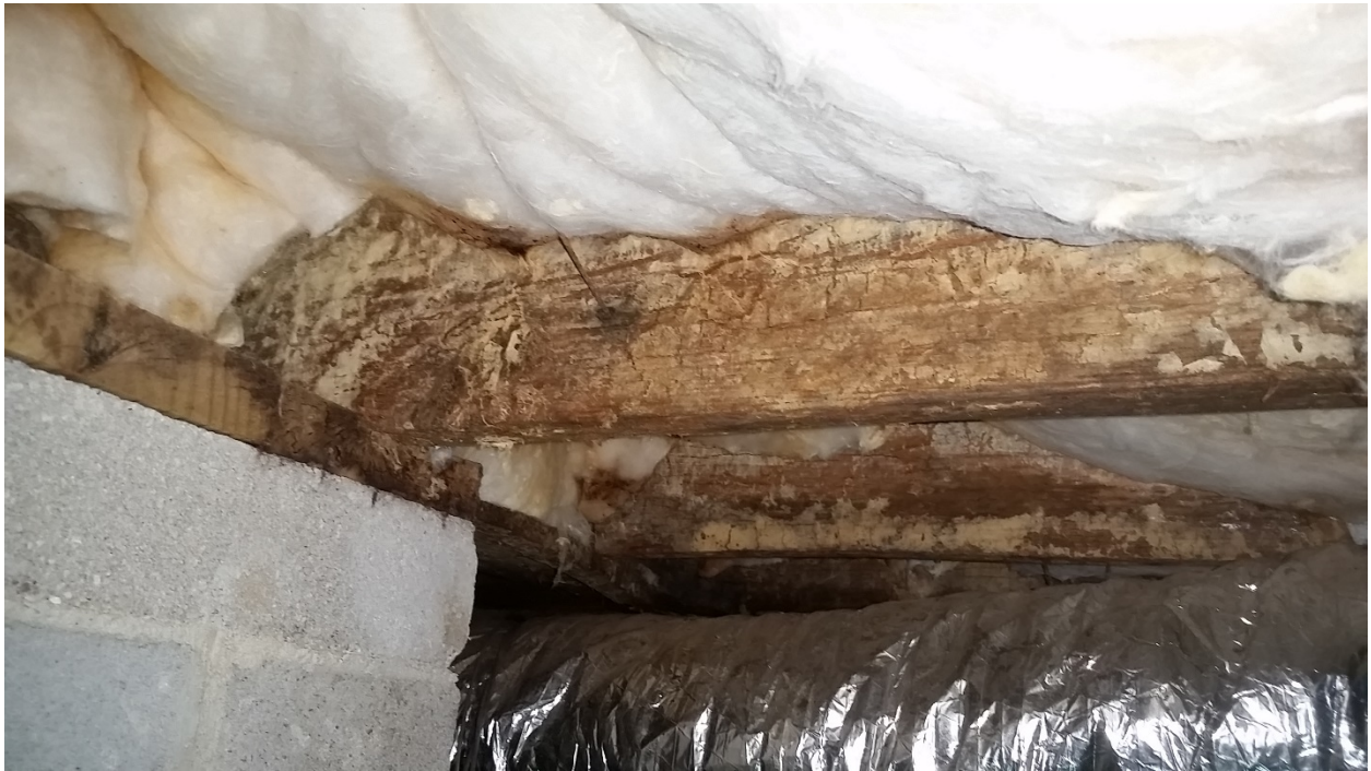
Darks Stained Deteriorated Floor Framing
