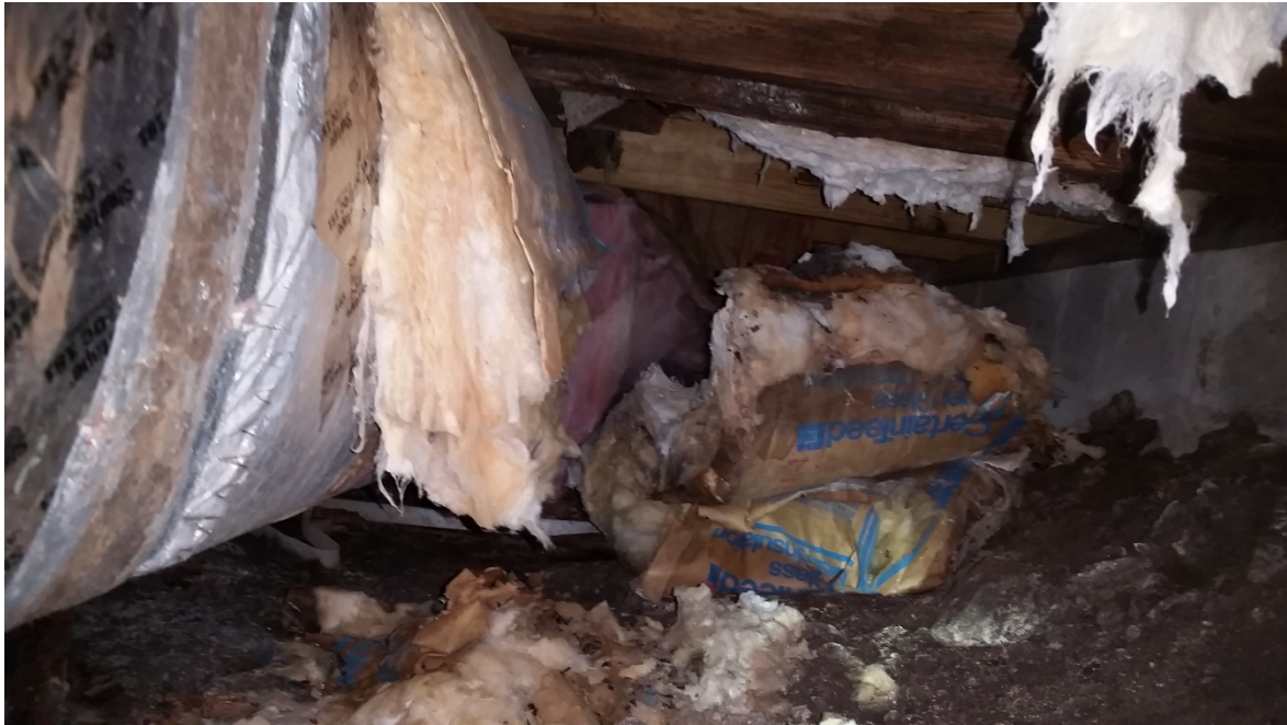
Fallen Insulation in Crawlspace
