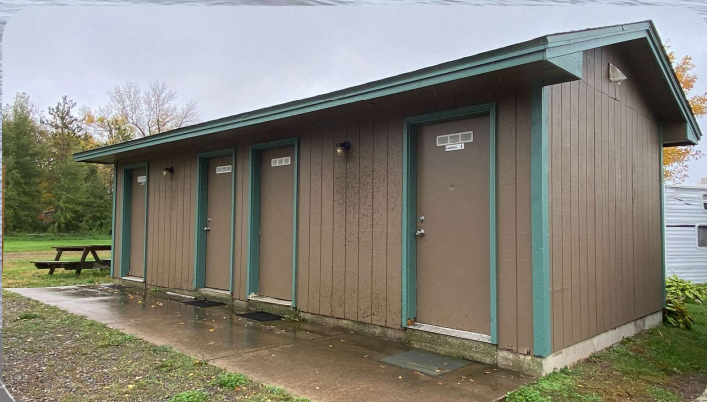
"East Side" Shower House
