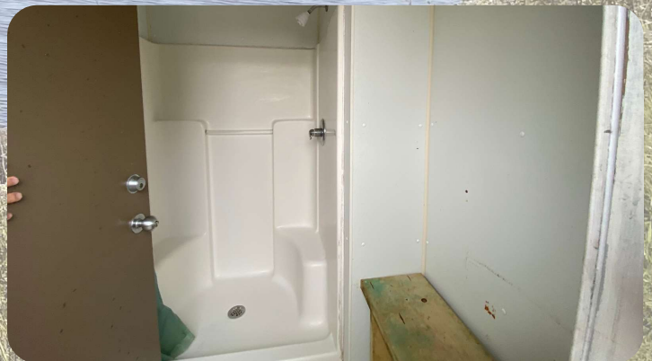
"East Side" Shower House
