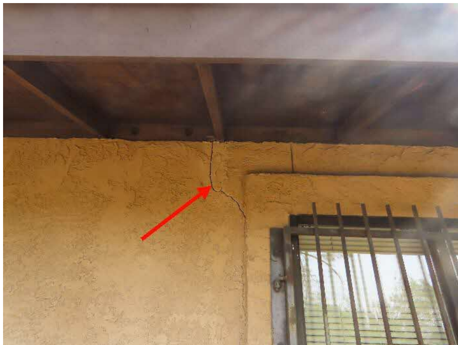
Photograph 22: A diagonal crack extends from the corner of a window opening.
