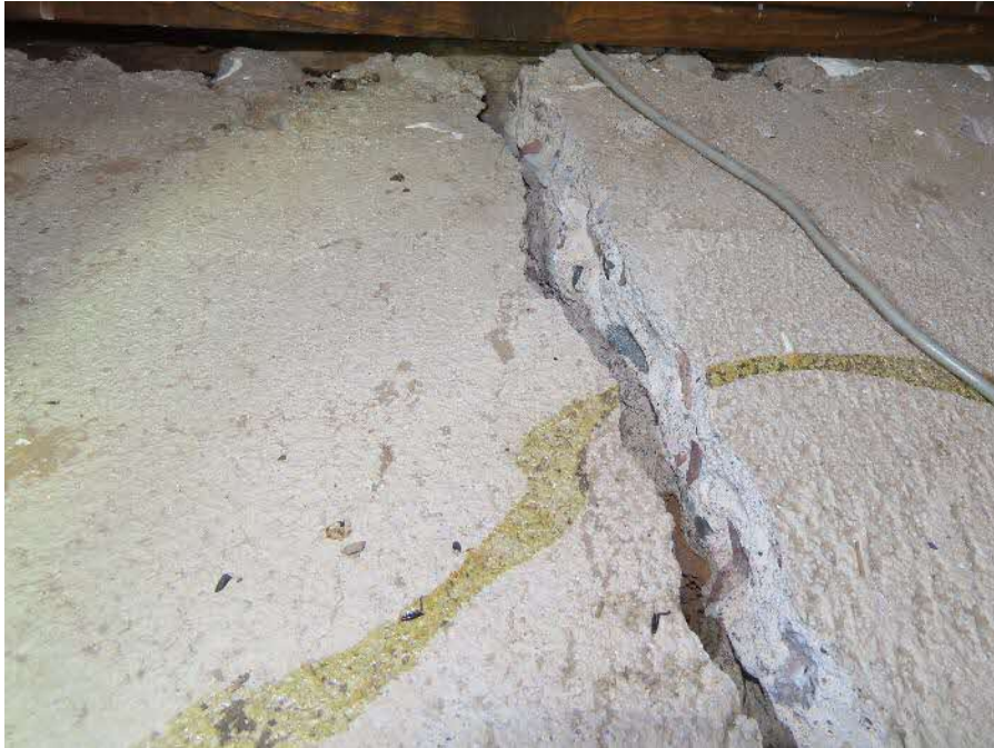
Photograph 7: The cracks has sharp, bright edges.
