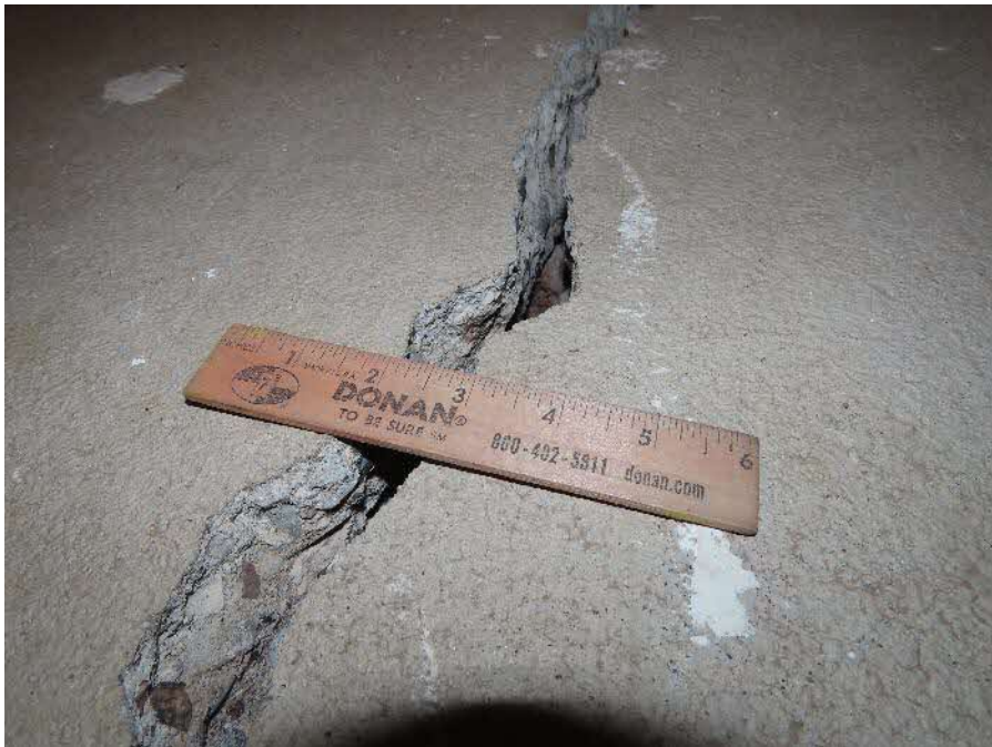
Photograph 6: The crack in the northwest bedroom floor slab.
