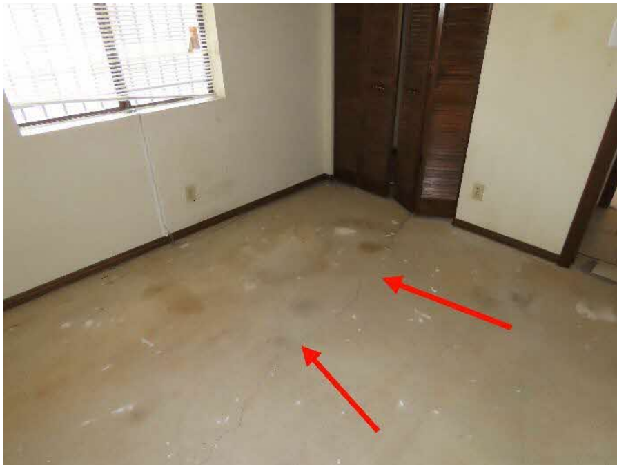
Photograph 8: The crack in the bedroom south of the northwest bedroom.
