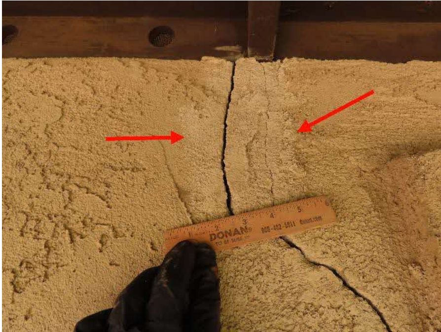
Photograph 23: The crack has rounded edges and is surrounded by paint that does not match the prevailing surface.
