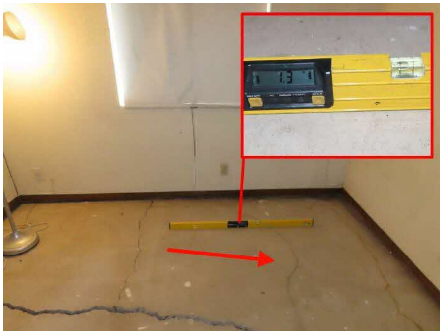
Photograph 14: A slope reading on the west side of the crack.
