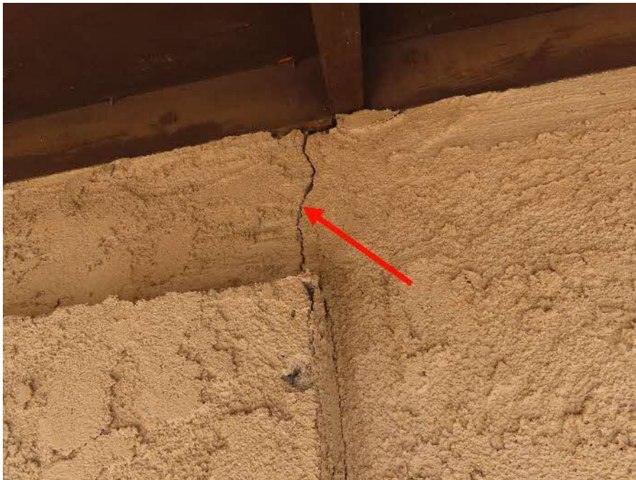
Photograph 20: A crack in stucco that extends from the corner of a window opening.
