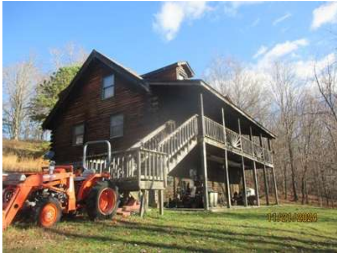
Main Structure Photo
