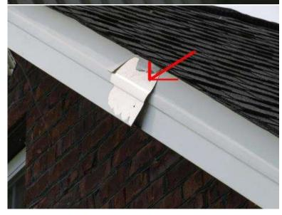
**Maintenance:** Soffit trim noted as loose and hanging in several locations around the structure at time of inspection. Suggest securing.
