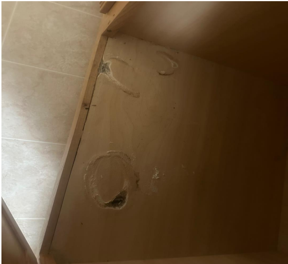
Water damage under bathroom sink.
