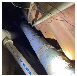
10.5.3 The ductwork is loose / poorly secured. A qualified HVAC contractor should repair as required to restore proper function. **(Crawlspace)**
