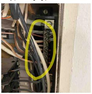
9.7.2 The sub-panel has double-tapped breaker(s). Recommend an electrician assess and correct as required for electrical safety. (Garage)
