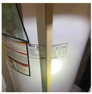
11.5.3 \* Water heater function not tested due to being turned off at the circuit breaker during the inspection. Recommend having this tested for functionality and correct connections at the use points. (Laundry area)
