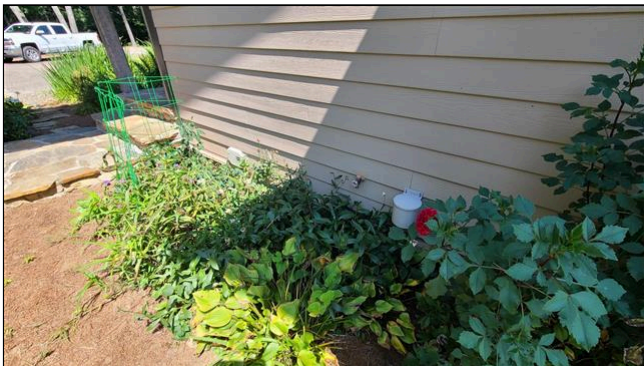
2.6 Item 5(Picture) front right corner
