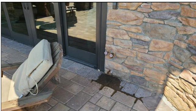
2.6 Item 7(Picture) rear left corner of the home
