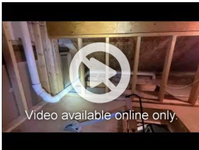
1.5 Item 1(Video) left side roof structure through primary bedroom closet
