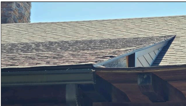
1.0 Item 7(Picture) front right corner by walkway
