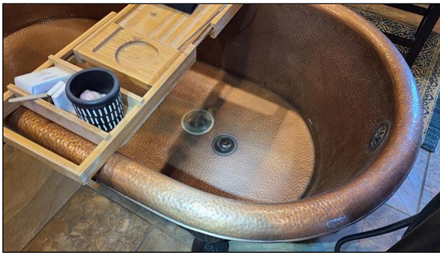
6.10 Item 1(Picture) visible debris in drain
