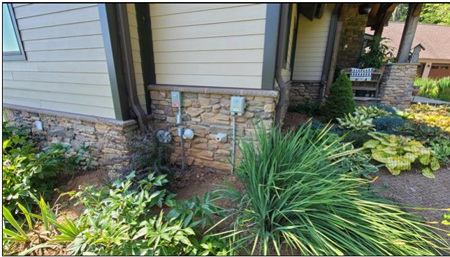
2.6 Item 1(Picture) front left corner of the home
