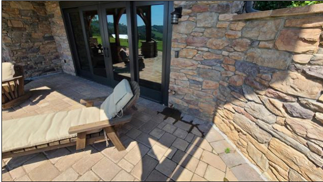
2.6 Item 3(Picture) rear left corner of the home - hot and cold water supply
