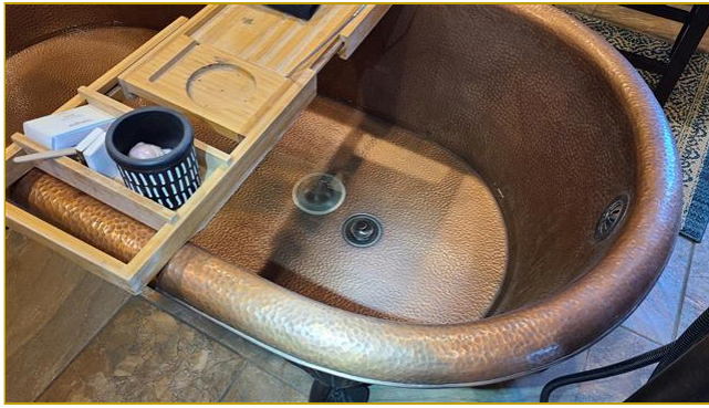
6.10 Item 1(Picture) visible debris in drain
