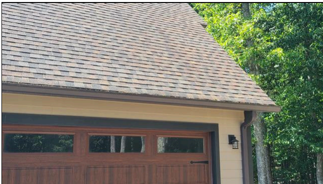
1.4 Item 2(Picture) front gutter for garage
