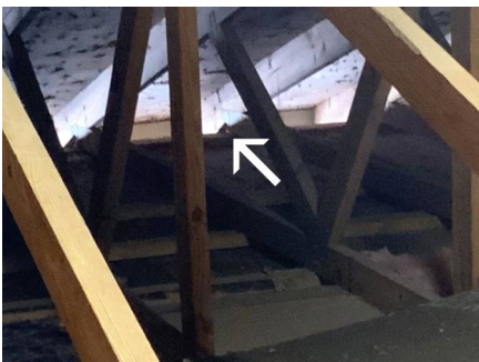
Roof to wall connection.
