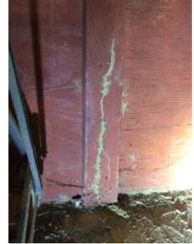
Termite activity attached shed
