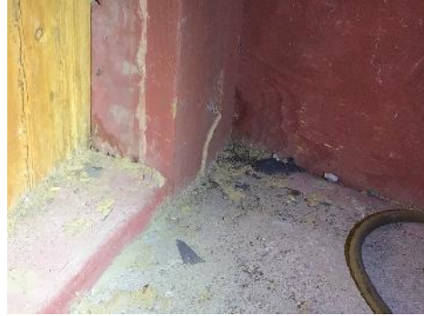
Termite activity attached shed
