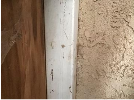
Termite activity attached shed
