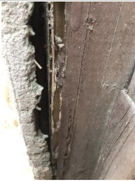
Termite activity attached shed
