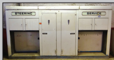
Front End Alignment Cabinet
