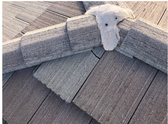
Broken mortar pack and tile
