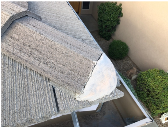
Broken mortar pack
