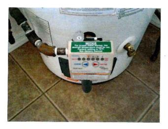
12. **Repair:** The closet unit is older and the life expectancy for the water heater is very limited. We recommend that a budget be made for the replacement of this unit in the very near future.
