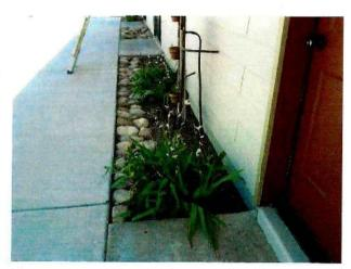
**Monitor:** The slope of the general site grading away from the structure was minimal at the front side area of the building. We recommend monitoring site drainage performance with repair as necessary.
