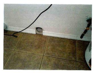
10. **Safety Concern:** The closet water heater combustion air supply vent was not present. Fuel burning appliances require oxygen carrying combustion air to operate safely. We recommend that a supply vent be installed in accordance with industry standards.
