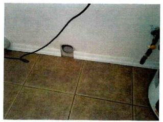
**Safety Concern:** The closet water heater combustion air supply vent was not present. Fuel burning appliances require oxygen carrying combustion air to operate safely. We recommend that a supply vent be installed in accordance with industry standards.
